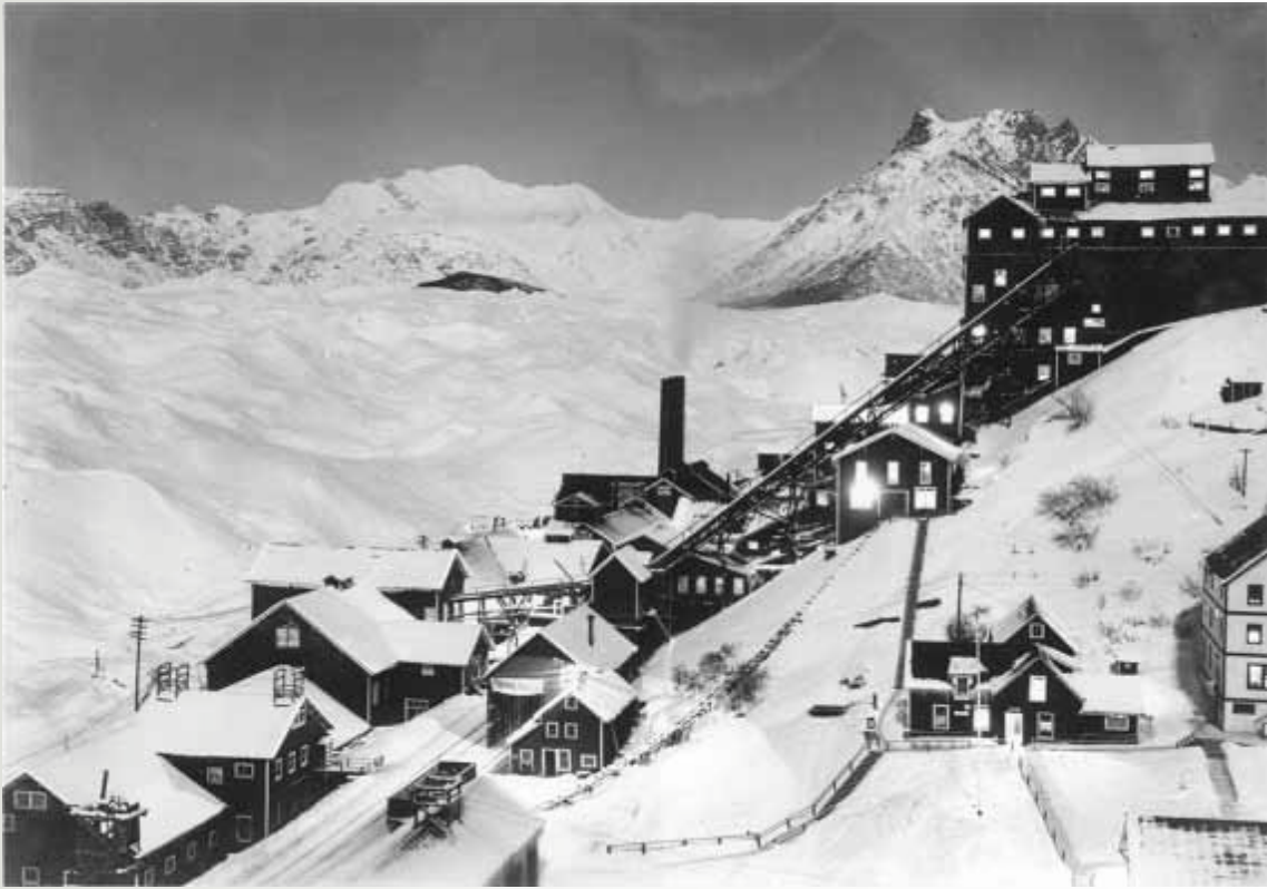
Image of Kennecott Mine power plant and facilities with the Root Glacier in the background, Kennecott Mines National Historic Landmark, Wrangell -St. Elias National Park and Preserve, McCarthy, Alaska. Photo and history of the mine available from www.nps.gov/wrst/images/20060705142735.JPG . Kennecott is considered the best example of early 20th Century copper mining.
