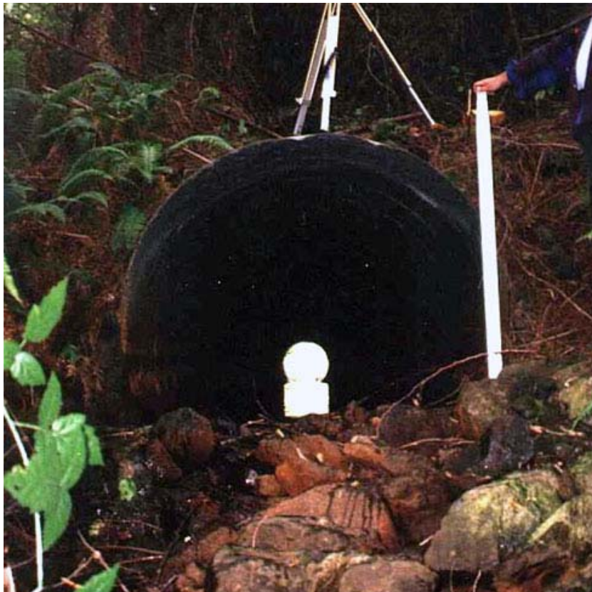
Figure 8.3 Pre-project barrier culvert (United States Forest Service 2006b)
