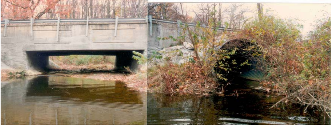
Figure 8.7 Downstream of pre-existing structure looking upstream
