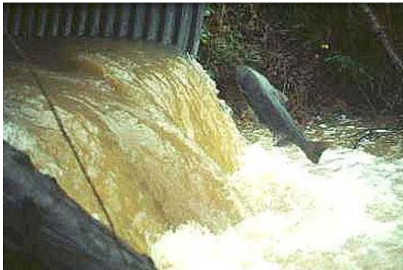
Figure 1.1 Scour downstream from culvert “perches” the barrel above the streambed, making it inaccessible to many fish species (United States Forest Service 2006b)
