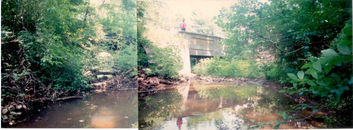
Figure 8.6 Upstream of pre-existing structure looking downstream
