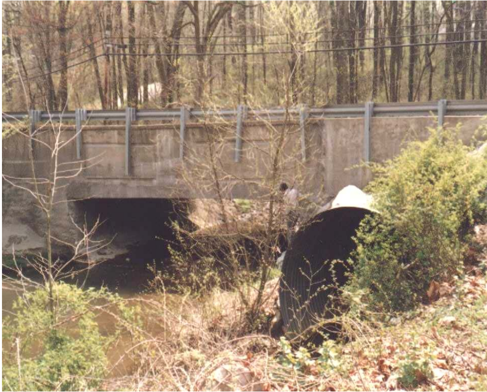
Figure 8.5 Pre-project channel condition (1992)
