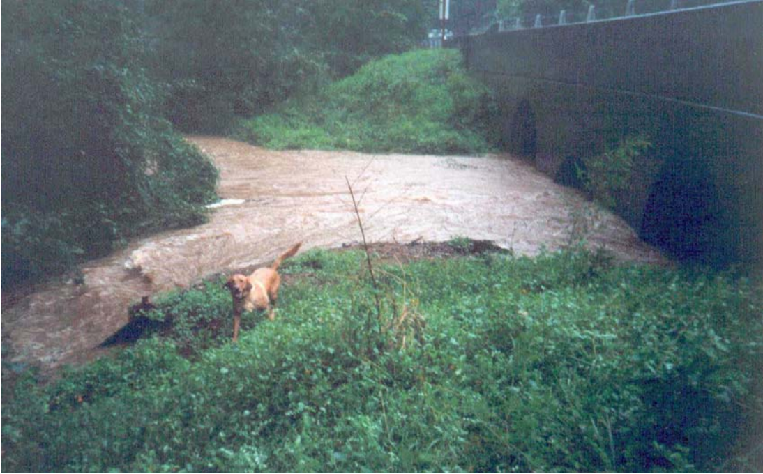
Figure 8.10 Upstream of current crossing during high-flow event
