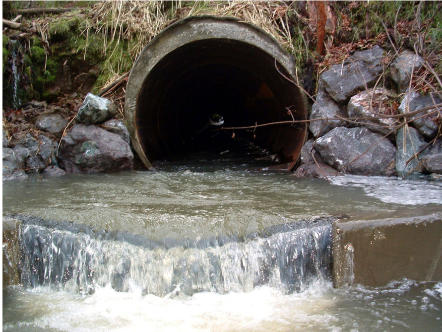
Figure 8.12 Downstream view of culvert retrofit, John Hatt Creek
