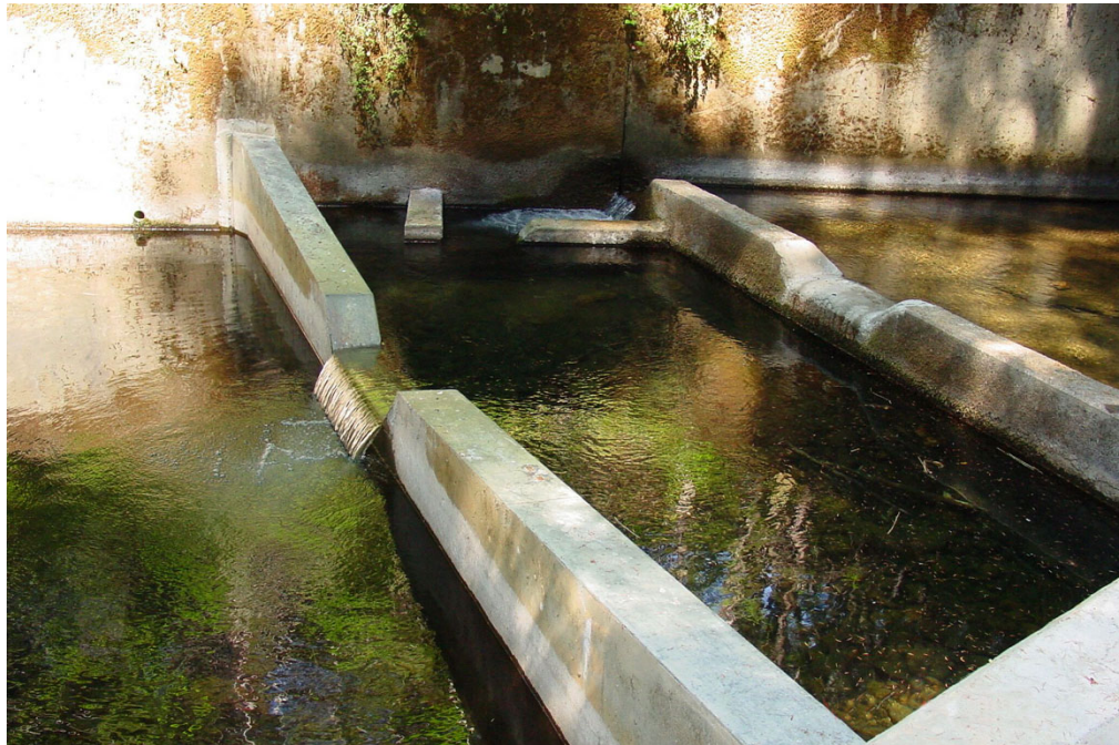
Figure 6.9 Notch weirs downstream of a culvert installation, acting to properly backwater the culvert, while maintaining manageable drops (United States Forest Service 2005)
