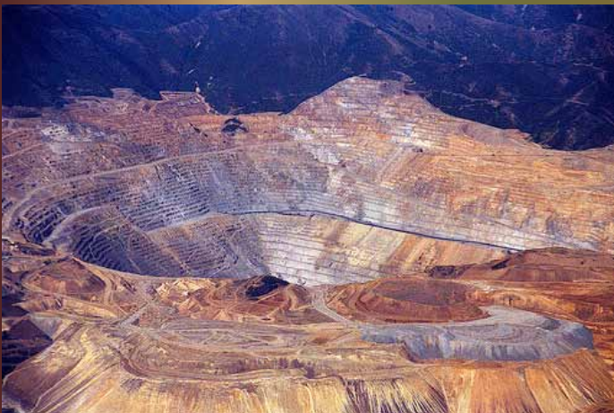
Figure 1. The Bingham Canyon Mine is the largest copper-sulfide mine in the world measuring 2.75 miles across the top and 0.75 miles deep. Acid waters, from the leaching of mine wastes, escaped the collection system and contaminated about 80 mi 2 of groundwater. See: http://www.epa.gov/region8/superfund/ut/kennecottsouth/ for more information.
