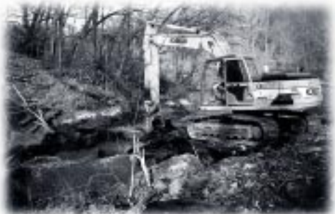
The Lititz Run Watershed Alliance in Pennsylvania removed an old dam to restore wildlife habitat and reduce thermal pollution in the stream.
