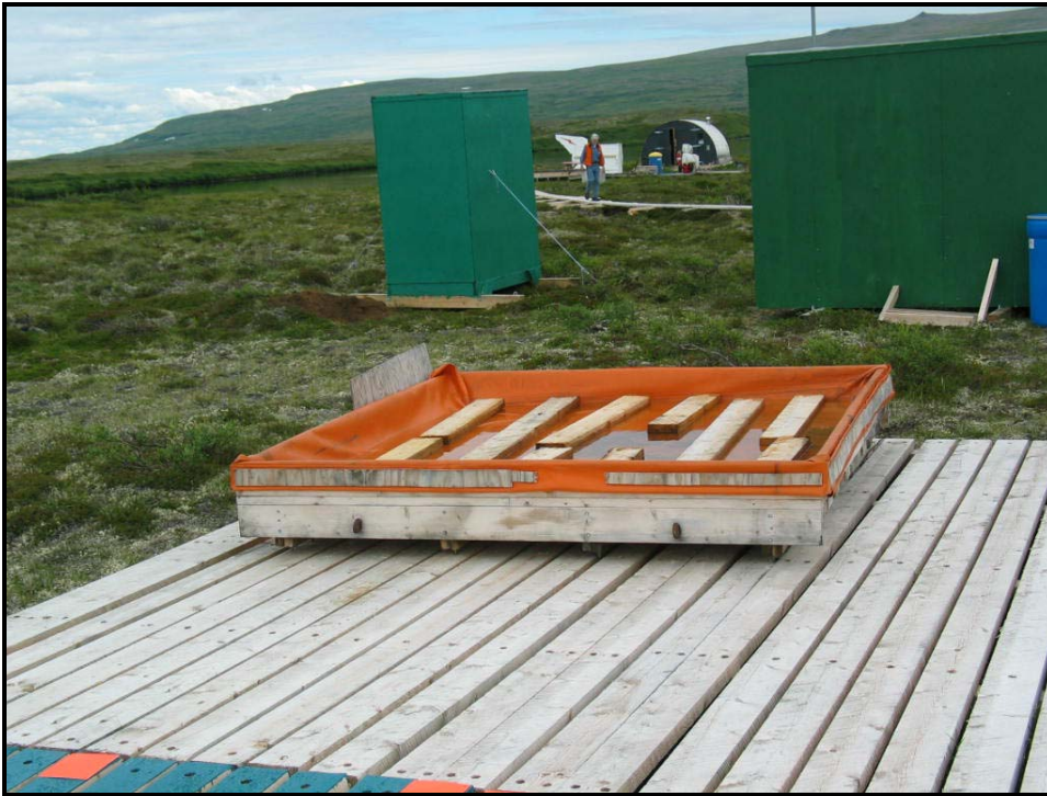
Photo #50. Lined containment for slinging fuel tanks in to 3,000 gallon fuel depot.
