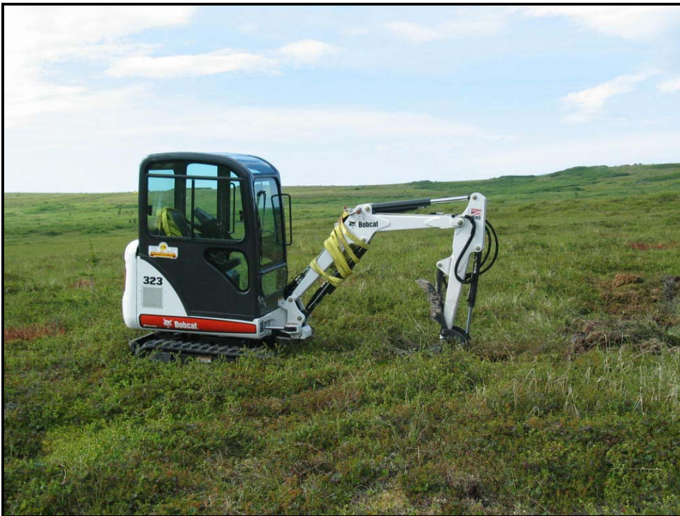
Photo #13. Small backhoe used for digging sumps. The backhoe is air lifted between sites.
