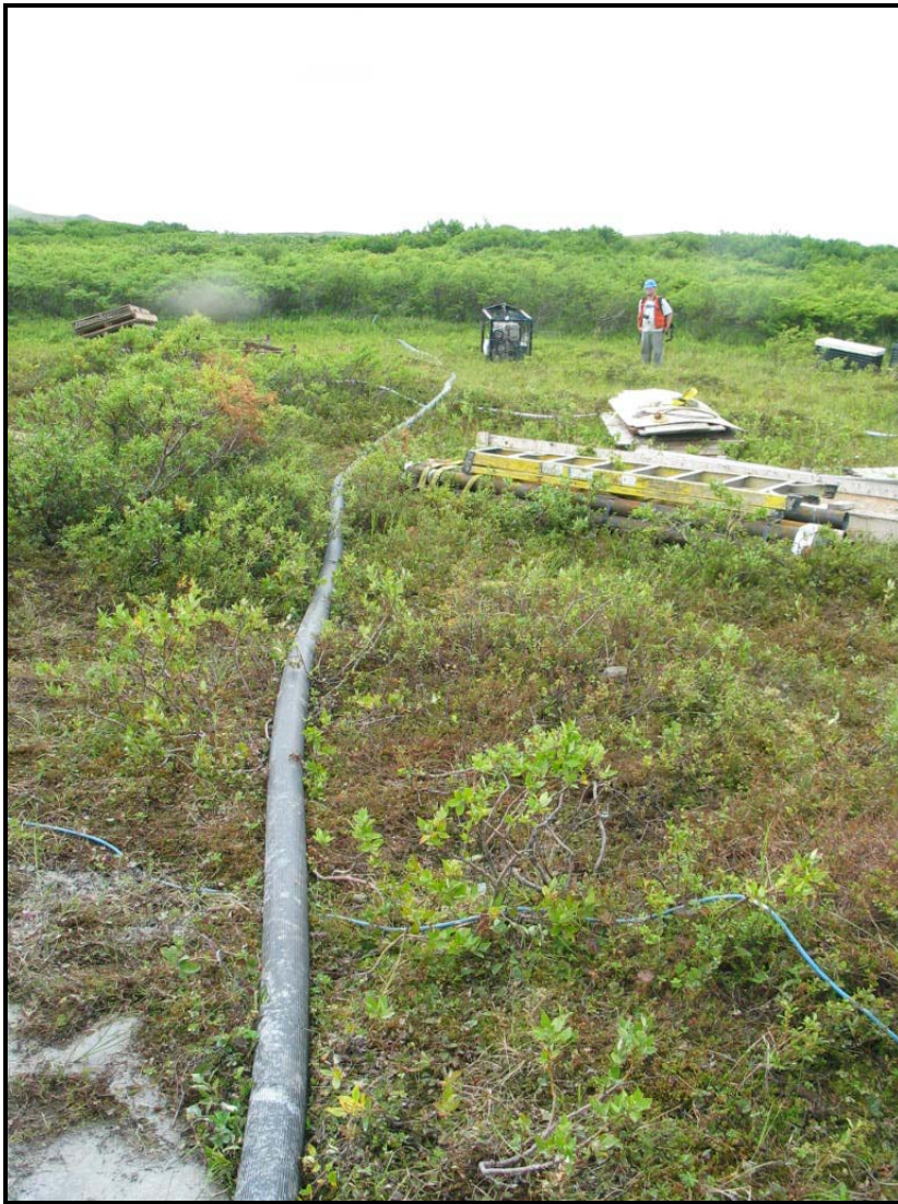
Photo #27. Hose carrying drilling fluids uphill to a topographic depression.
