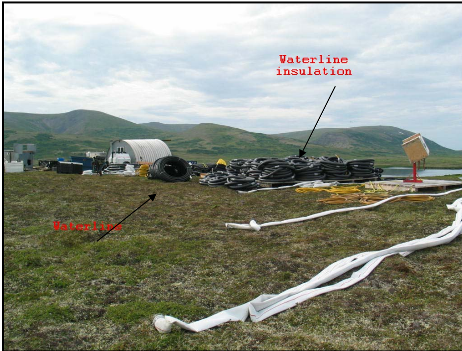
Photo #70. Waterline storage area.
