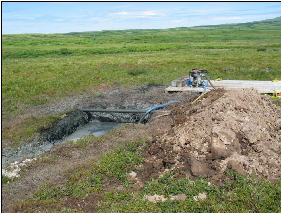
Photo #19. Sump at drill #6.
