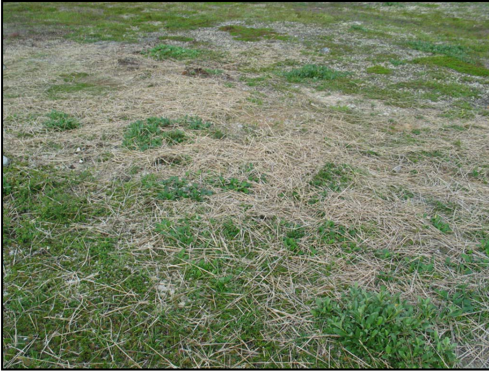
Photo #39. Reclamation at DDH 7364. Site has been treated with straw to prevent erosion, and seeded with grass. Note new vegetation.
