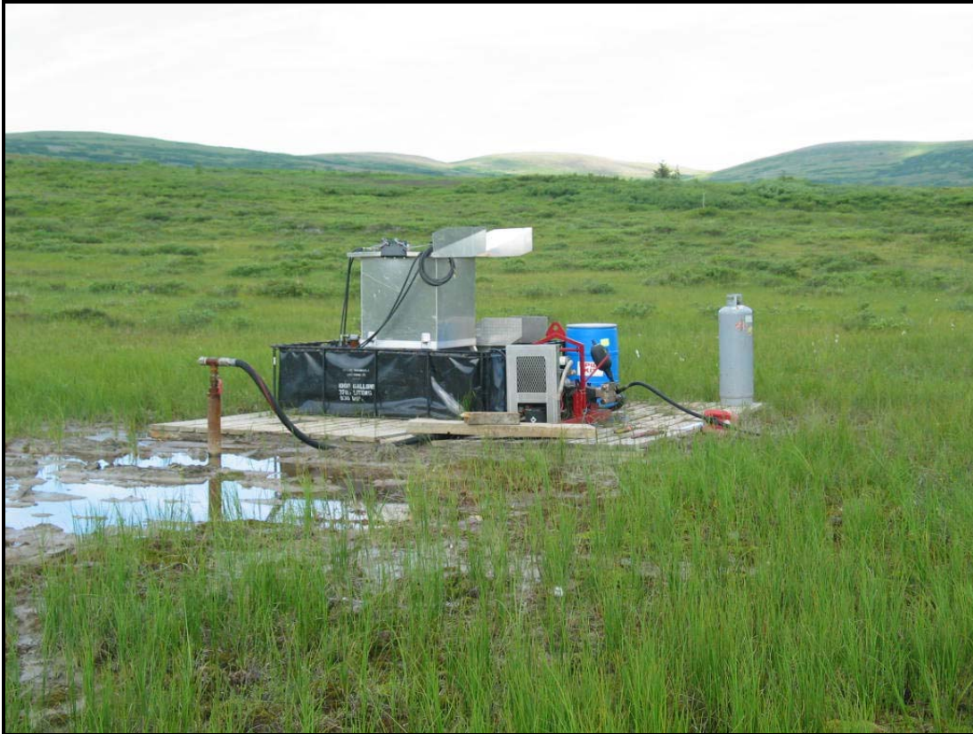
Photo #56. Water pumping facility taking water from a recently drilled hole.
