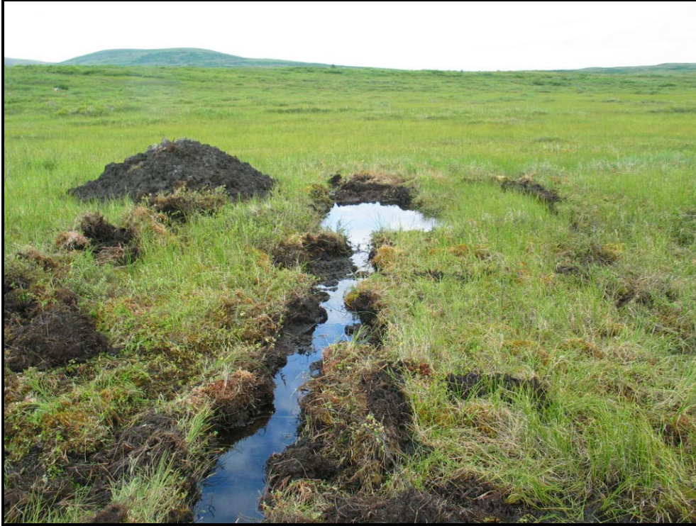
Photo #12. Drainage ditch and sump at new drill site.
