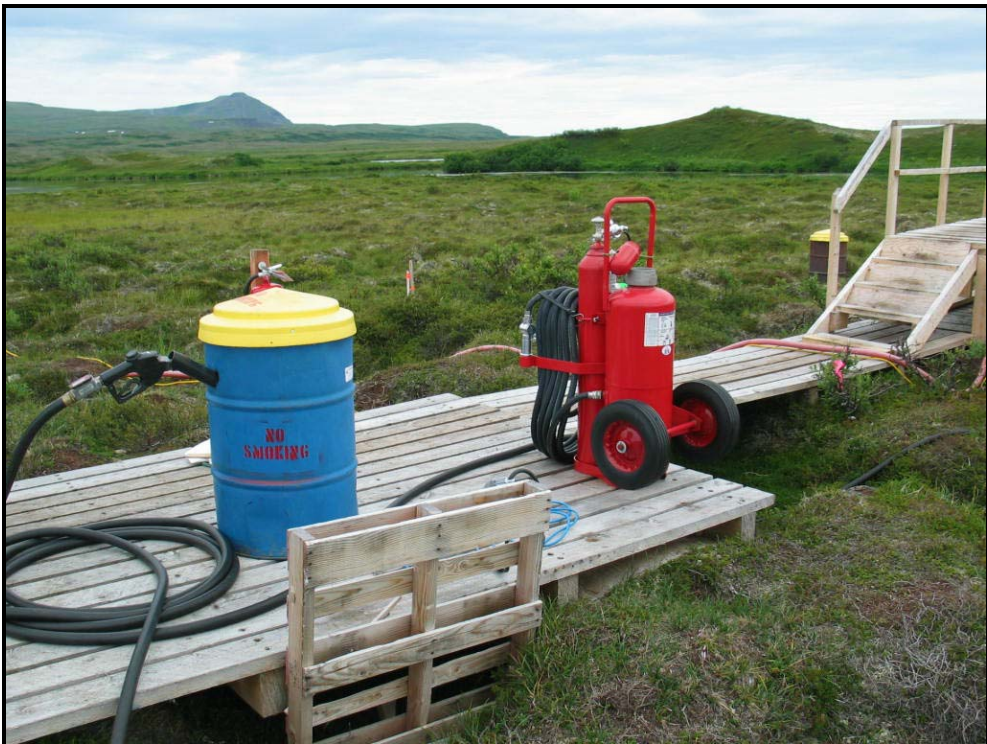
Photo #53. Large fire extinguisher at Big Wiggly fuel storage facility.
