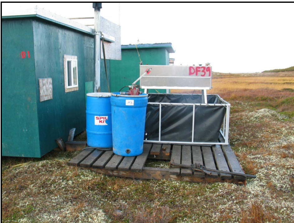
Photo #2. Fuel tank and containment for crew quarters on drill site.
