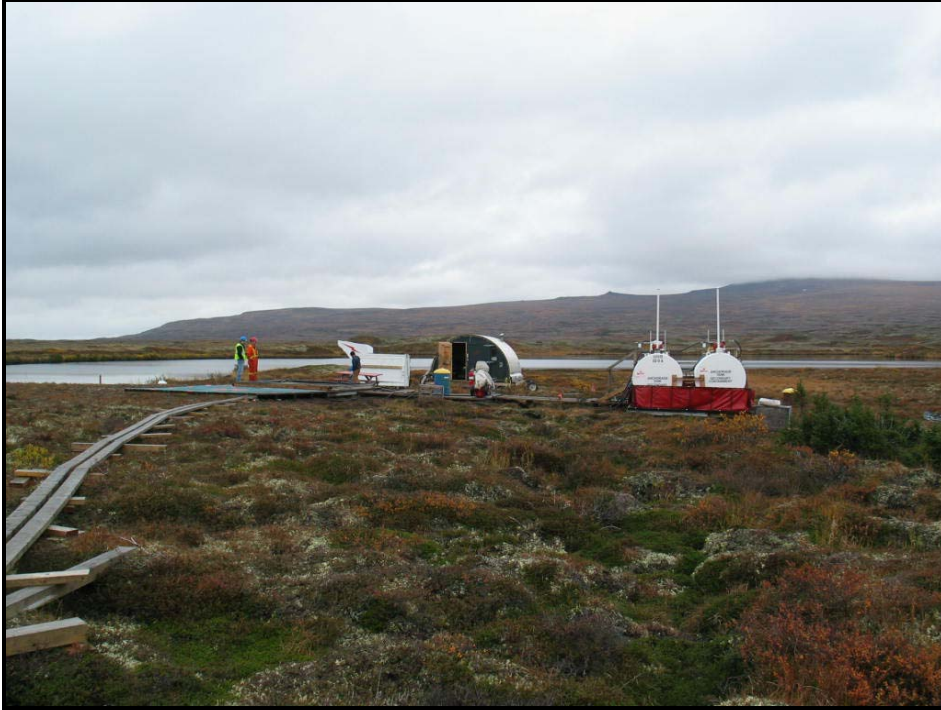
Photo #13. Big Wiggley fuel storage facility – 2,000 gallon storage containment. Boardwalk is for tundra protection.
