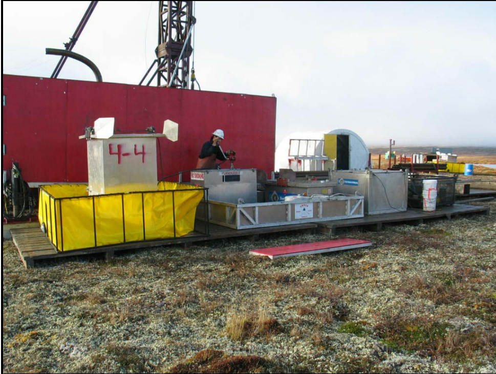
Photo #1. A drill crewmember pumps fuel from 118 gallon aluminum slinging tank into main fuel storage tank at drill #4. Note that the sling tank is in a metal containment. The main fuel tank is in the yellow plastic containment.
