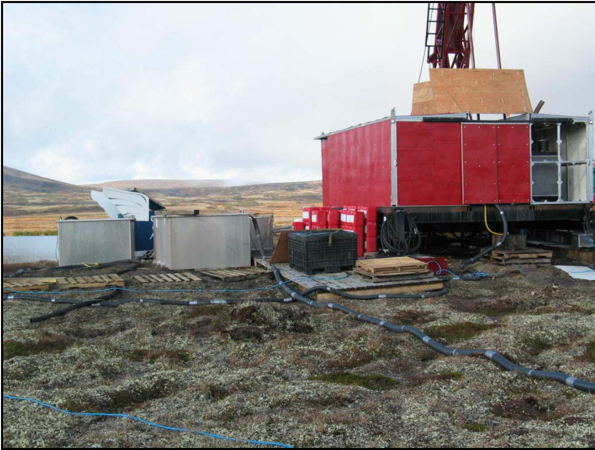
Photo #11. Extra tanks required for recirculating drilling fluids at drill #1.
