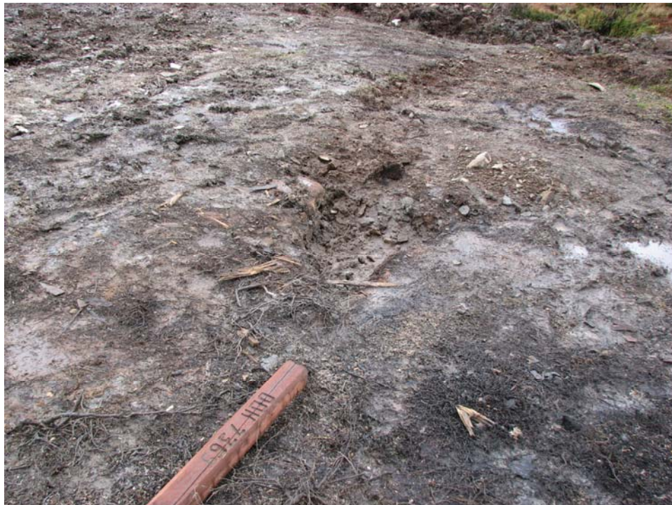
Photograph No. 4: Drill Site No. 7369 Well casing cut off below ground. Reclamation work started.
