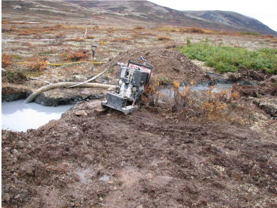
Photograph No. 1: Drill Site No.7384 trench and sump pit.
