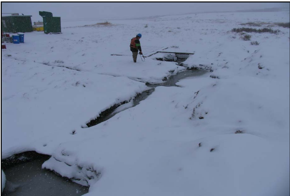
Picture 4 - DDH 077368 Sump
