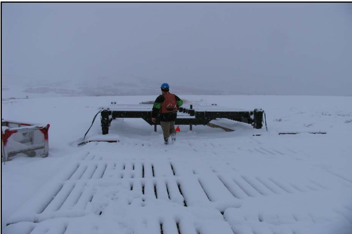
Picture 13 (Next Site of Drill Rig 2)
