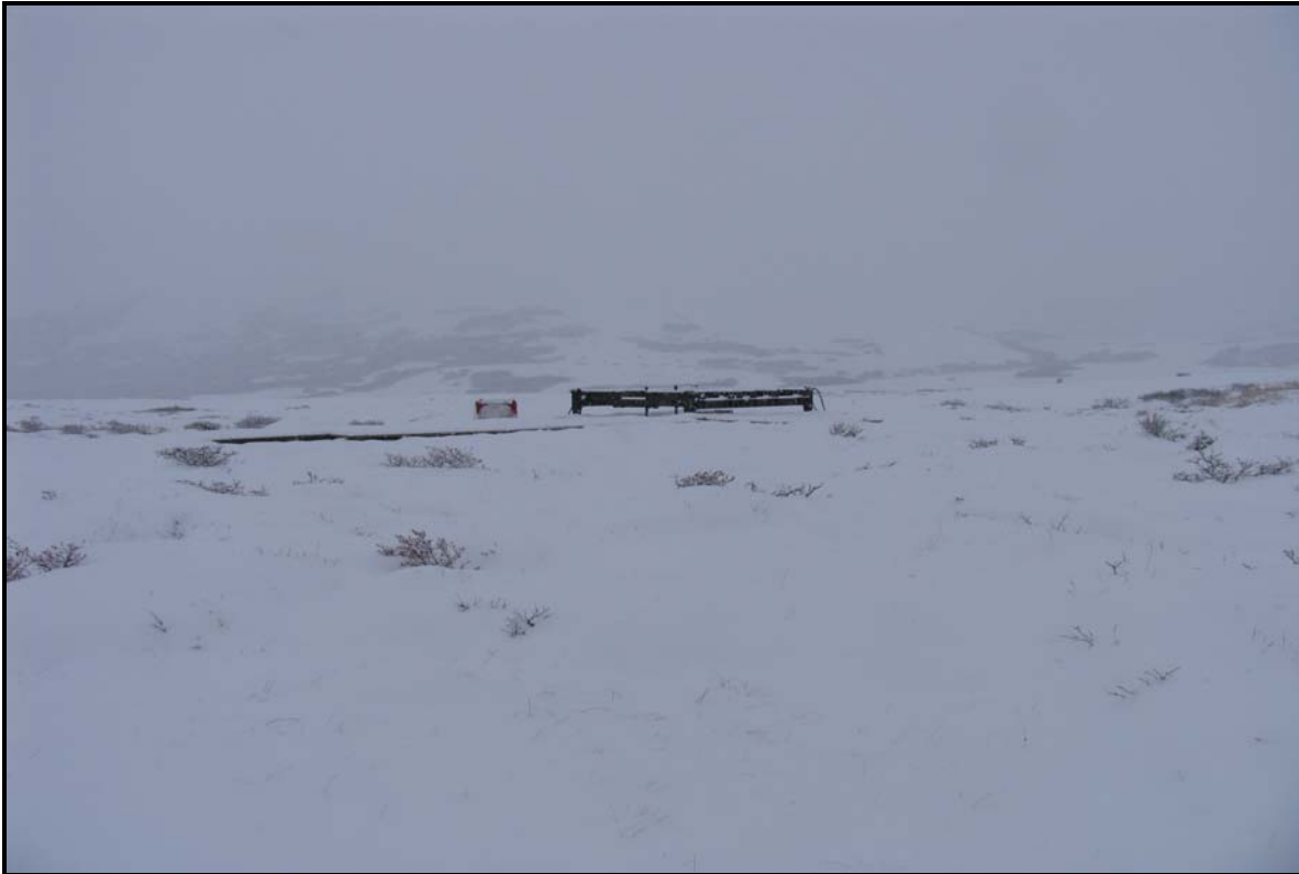
Picture 12 (Next Site Drill Rig 2)
