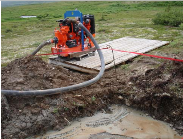
Figure 7. Godwin pump for drilling fluids at drill rig 3.
