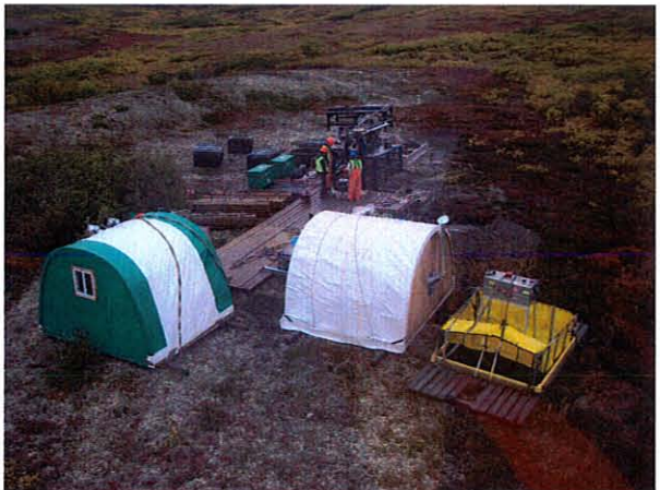
Figure 6. Drill rig 9, geotechnical drill hole.
