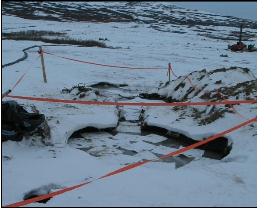
Photo #19. Sorbent pads on sump pits at drill #4.
