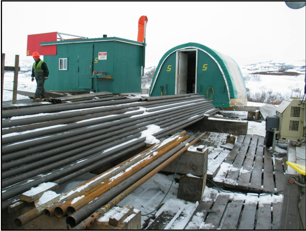
Photo #25. Drill rods at rig #5.
