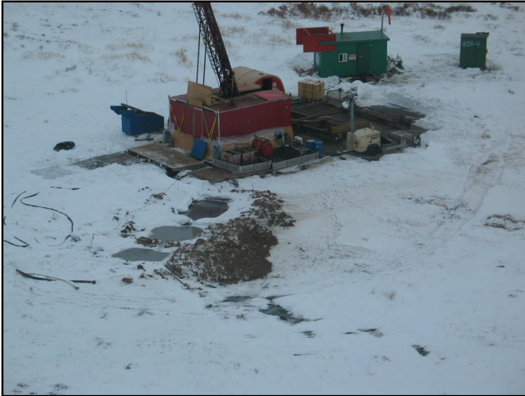
Photo #15. Drill #3, sump pits and drilling discharge.
