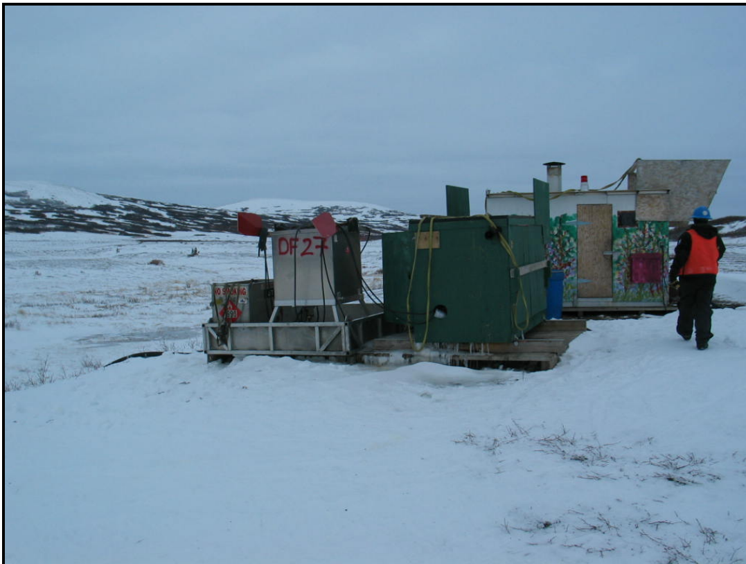
Photo #16. Water pump for drill #3.
